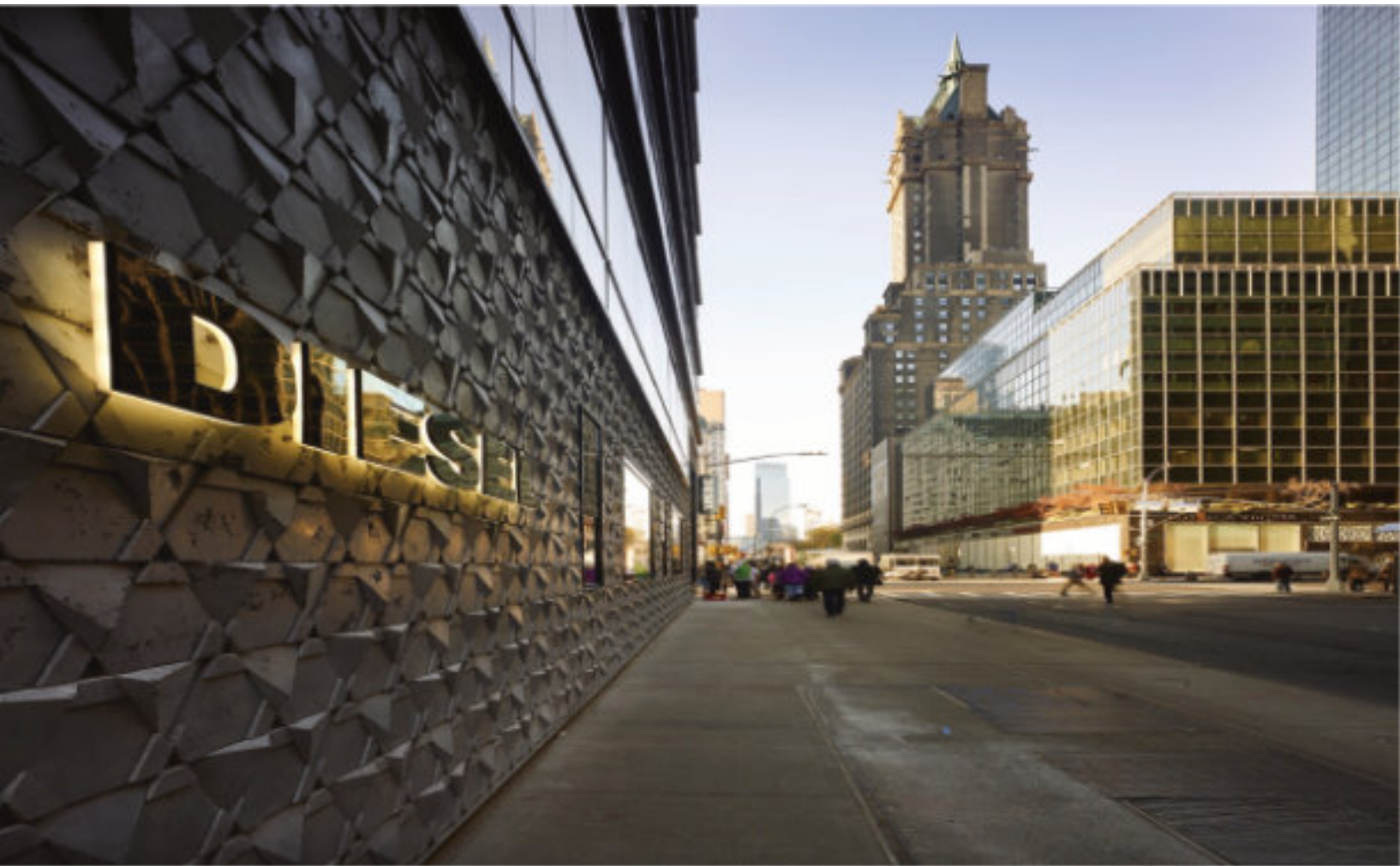
Diesel store, NY, UHPC "vibrato"
